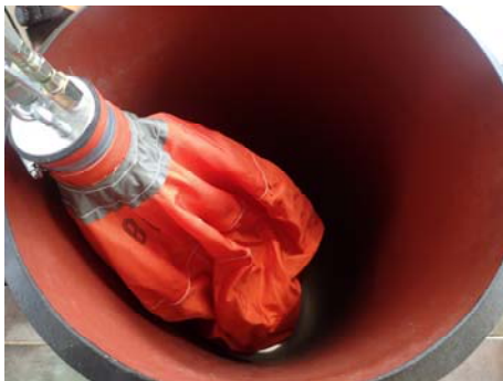
Figure 3 – Deployed Dual Gas Bag into pipe spool
