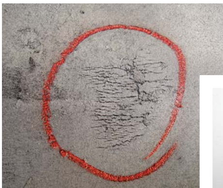
Axially-oriented crack colony
