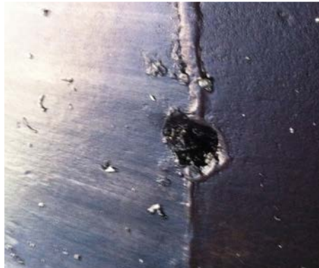
Girth weld defect
