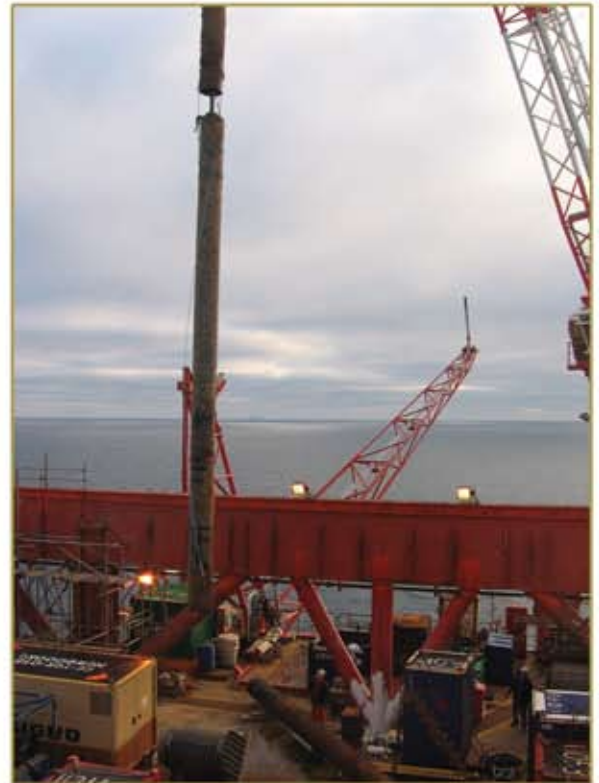
24" Internal Lifting Tool - Caisson Removal
